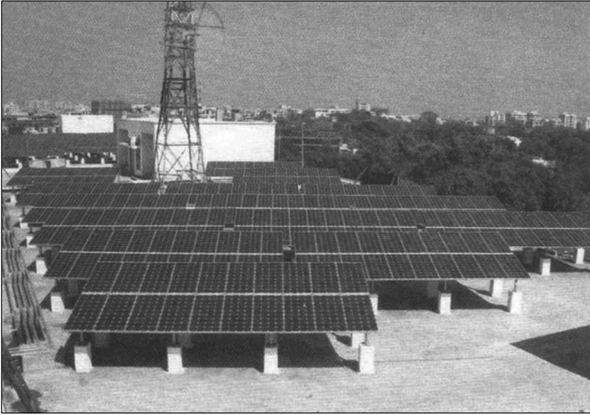
100 kWp SPV Grid Interactive Power Plant at APTRANSCO, Hyderabad
