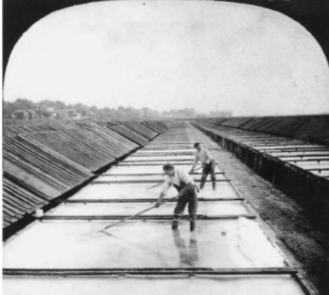
*Half of an 1890 stereo card of the Onondaga saltworks showing salt being raked from solar evaporation vats with rolling roofs of a design copied from the Cape Cod saltworks. Onondaga County Salt Museum, Liverpool, New York*
